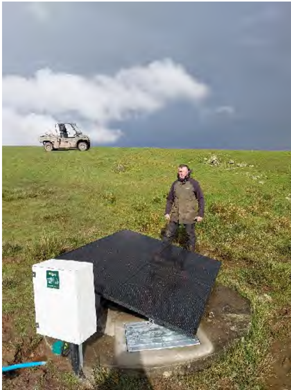
Solar powered pump for livestock watering
